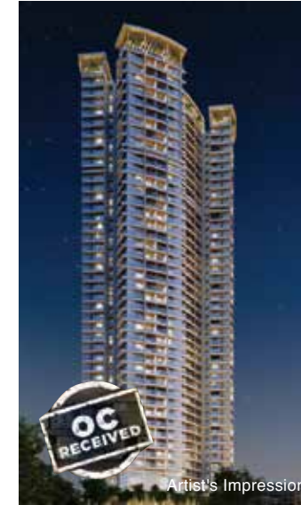
JP DECKS GOREGAON EAST
