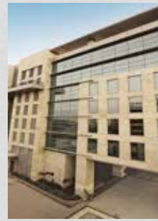
KALPATARU SQUARE ANDHERI (E)
