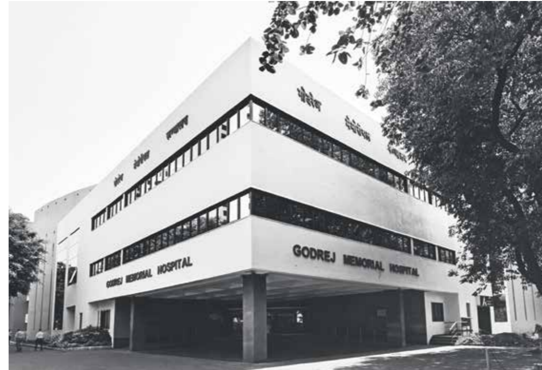
Godrej Memorial Hospital
