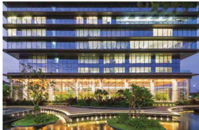
Actual Photograph of Godrej One Landscaping
