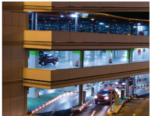
9 level podium parking
