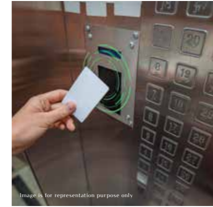
Access controlled Elevators
