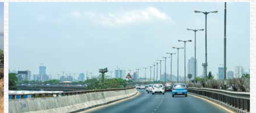
45 Minutes To South Mumbai Via Eastern Exp. Highway & E. Freeway.
