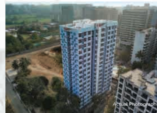
PLATINUM TOWER - 1 ANDHERI (W)
