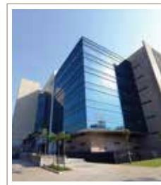
2013 – KALPATARU PRIME, THANE, One of Thane's prime commercial property
